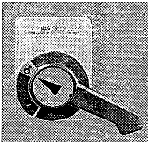
Isolator in OFF position.
